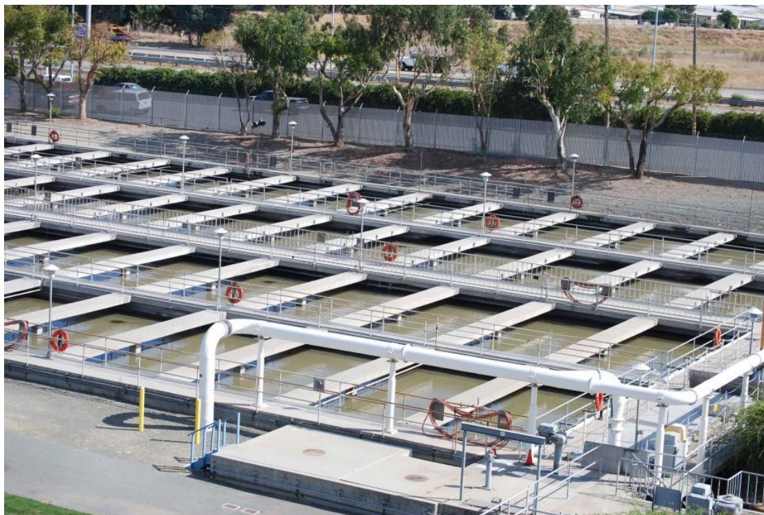
Part of a wastewater treatment plant in Contra Costa County. (Image: File)
